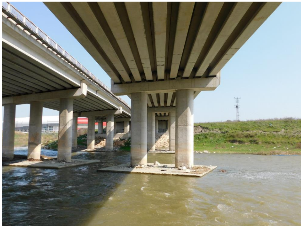
Figure 5-13 Overall view from under Bridge 2
