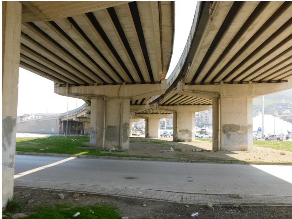
Figure 5-33 View under Bridge 3, showing 11 precast I-girders per span for each bridge
