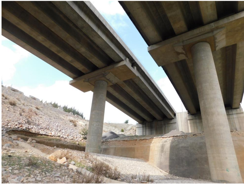
(a) Looking toward abutments of adjacent bridges
