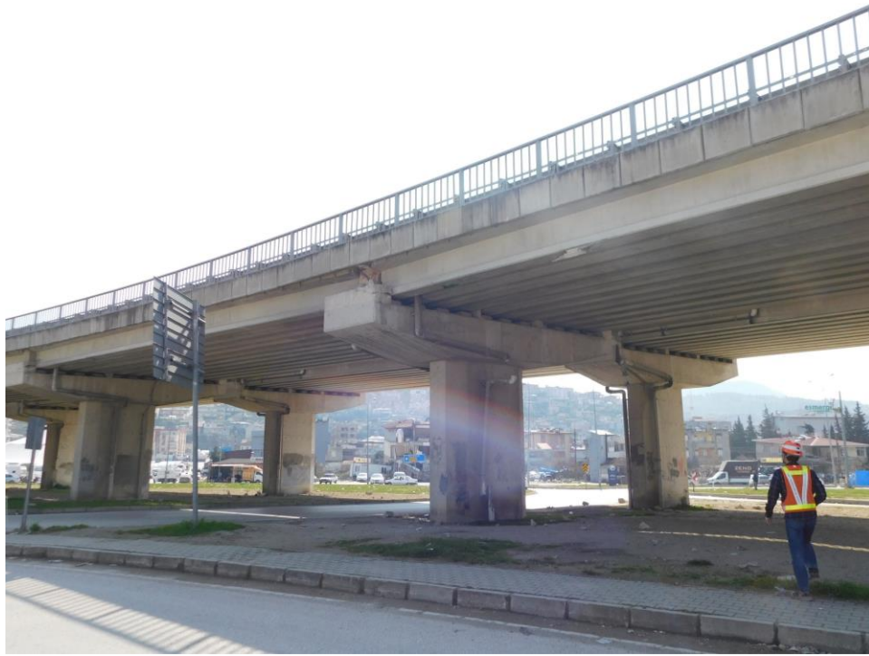
Figure 5-32 Overall view of Bridge 3
