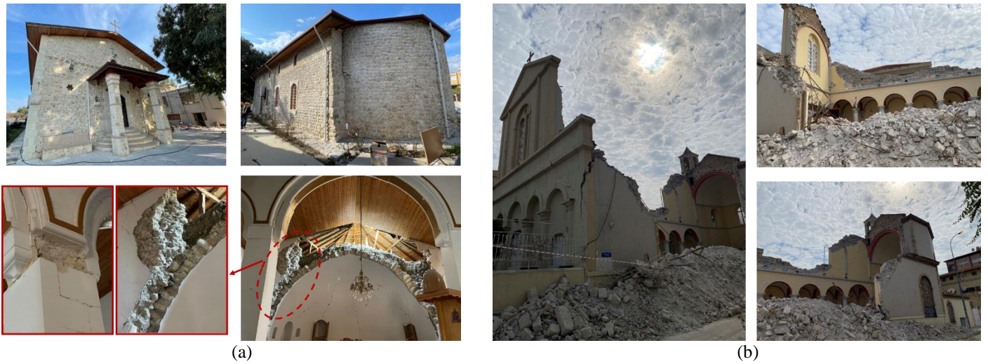
Figure 7-3 Damage of Churches (a) St. Ilyas Church in Samandagi, Antakya, (b) Roman Catholic Church in Iskenderun
