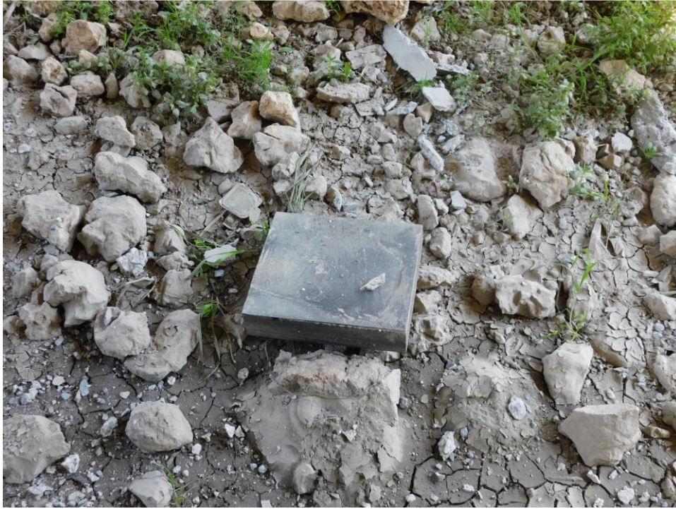
Figure 5-17 Rubber bearing pad on ground; one of many, Bridge 2
