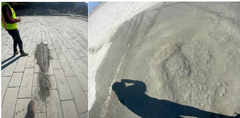
Figure 3-4 Liquefaction manifestations (sand boils) on Ataturk Boulevard near Ataturk (~ 36°35'29.50"N/ 36° 10'20.23"E)
