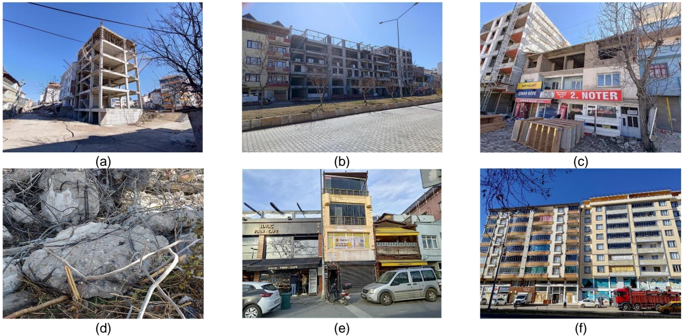
Figure 4-2 (a) and (b) two buildings with different construction practices, (c) a building with an added third story, (d) poor concrete and plain reinforcement, (e) and (f) no separation between buildings.
