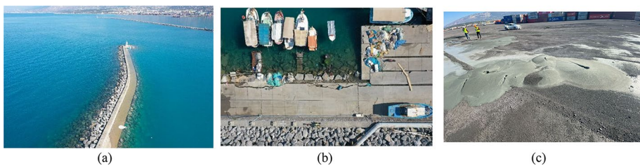
Fig. 8 Ground settlements and lateral deformations on Iskenderun dock (~36°35'40.67"N/36° 10'38.69"E): a ground subsidence at the pier and the lighthouse; b ground subsidence at the dock; c free field sand boils at the port
