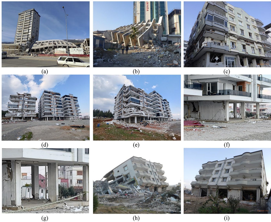
Fig. 17 a and b lie-down collapsed buildings, c a building with pancaked third story, d and e three similar buildings with different damage states, f close-up photograph of the first story of the right building, g bi-directional and one-directional plastic hinges, h and i a knee-down collapsed building
