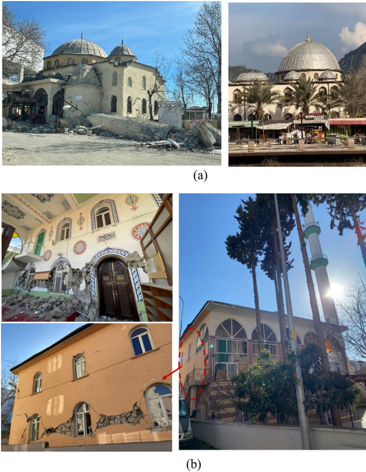
Fig. 36 Damage of mosques a Haci Murat Mosque in Kahramanmaraş, b Merkez Cumhuriyet Mosque in Pazarcik
