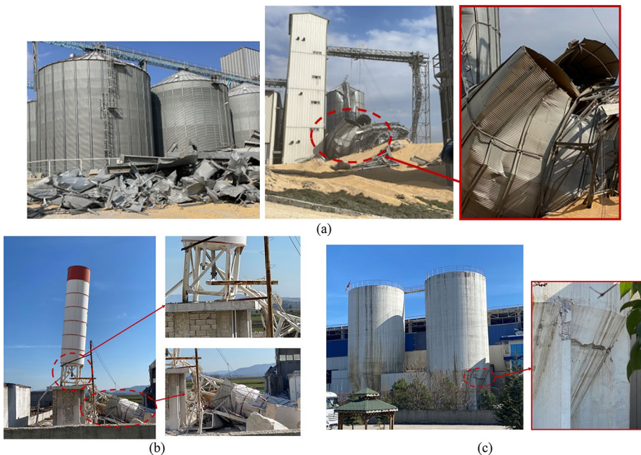
Fig. 34 Damage of silos a corn silos, b total collapse of a slender metal silo due to brittle welded connection, c concrete spalling on silos
