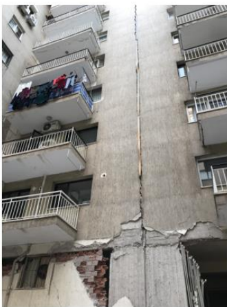
Figure 15. Inadequate Earthquake Joints in Bayraklı district of İzmir, Turkey
