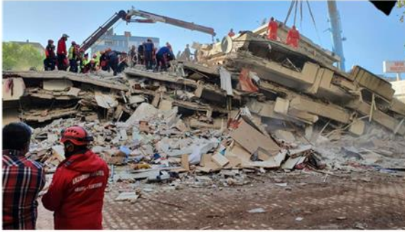
Figure 13. Damage due to Weak Column Strong Beam (WCSB) Ratio
