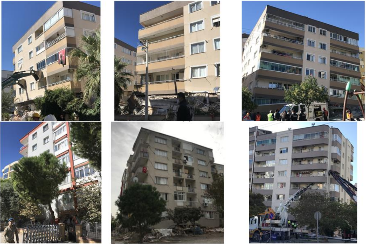
Figure 11. Partially collapsed buildings due to the soft story mechanism at the first floor in Bornova district in İzmir, Turkey
