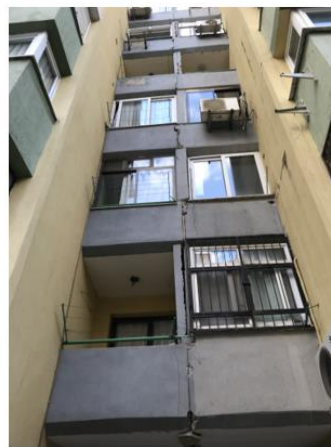
Figure 15. Inadequate Earthquake Joints in Bayraklı district of İzmir, Turkey
