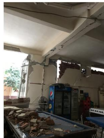
Figure 15. Inadequate Earthquake Joints in Bayraklı district of İzmir, Turkey
