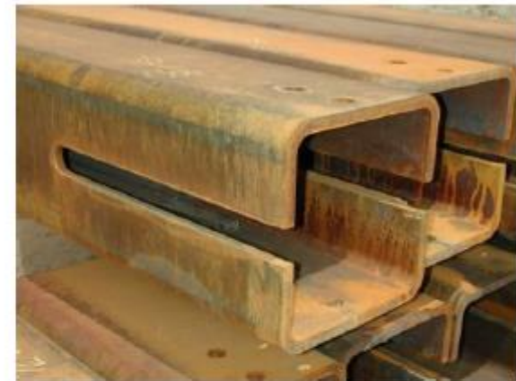
Fig. C-D3.4. Net area through slot for single gusset plate.
