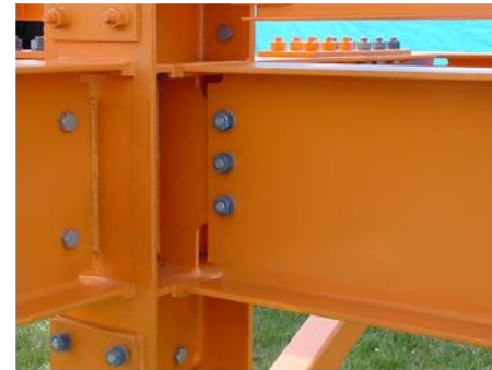
Flange Welded Moment Connection
