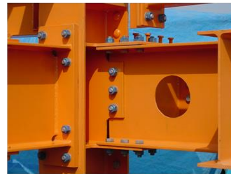
Bolted Moment Connection
