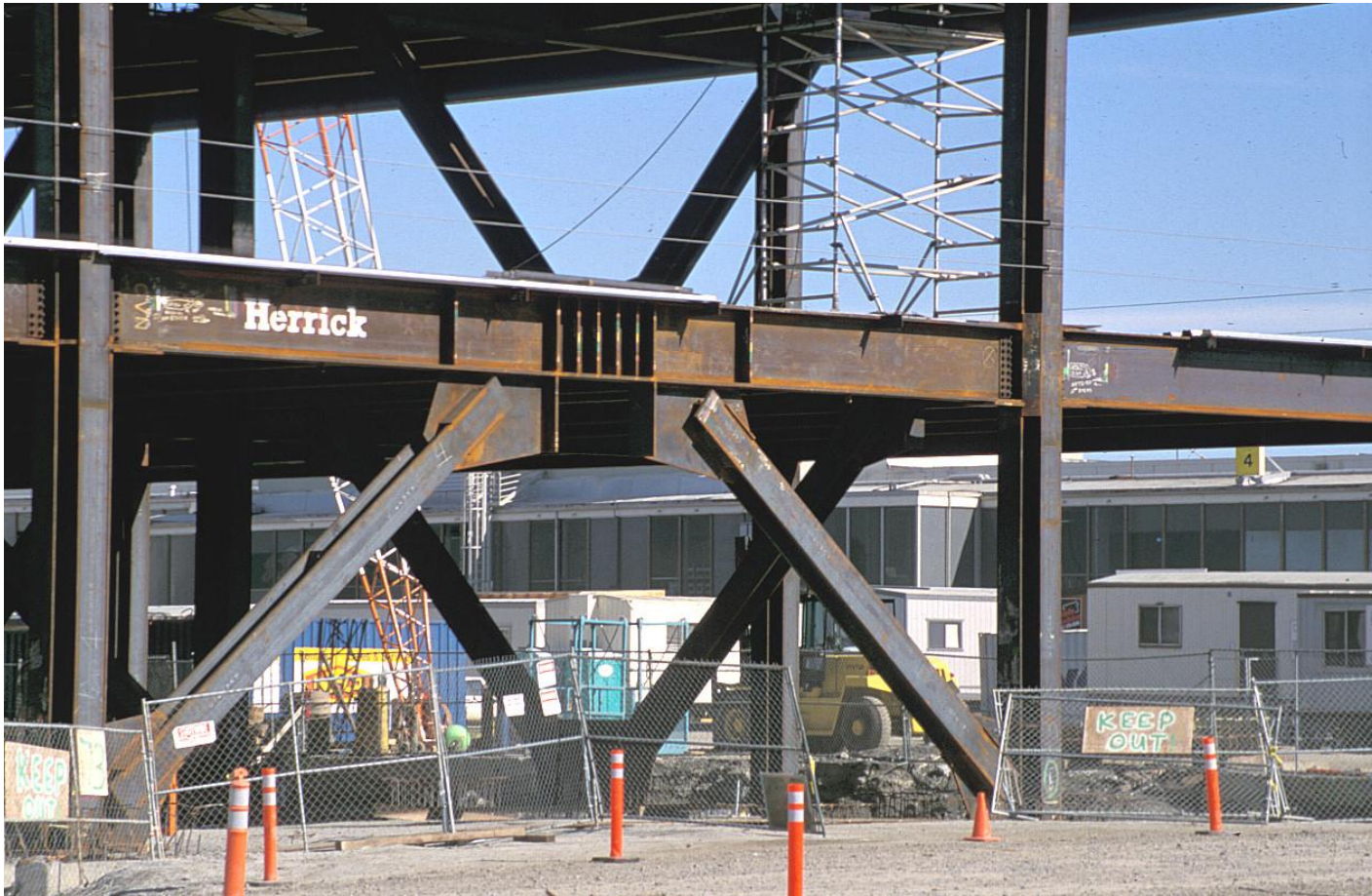
Link beams at beam mid-spans, San Francisco Airport
